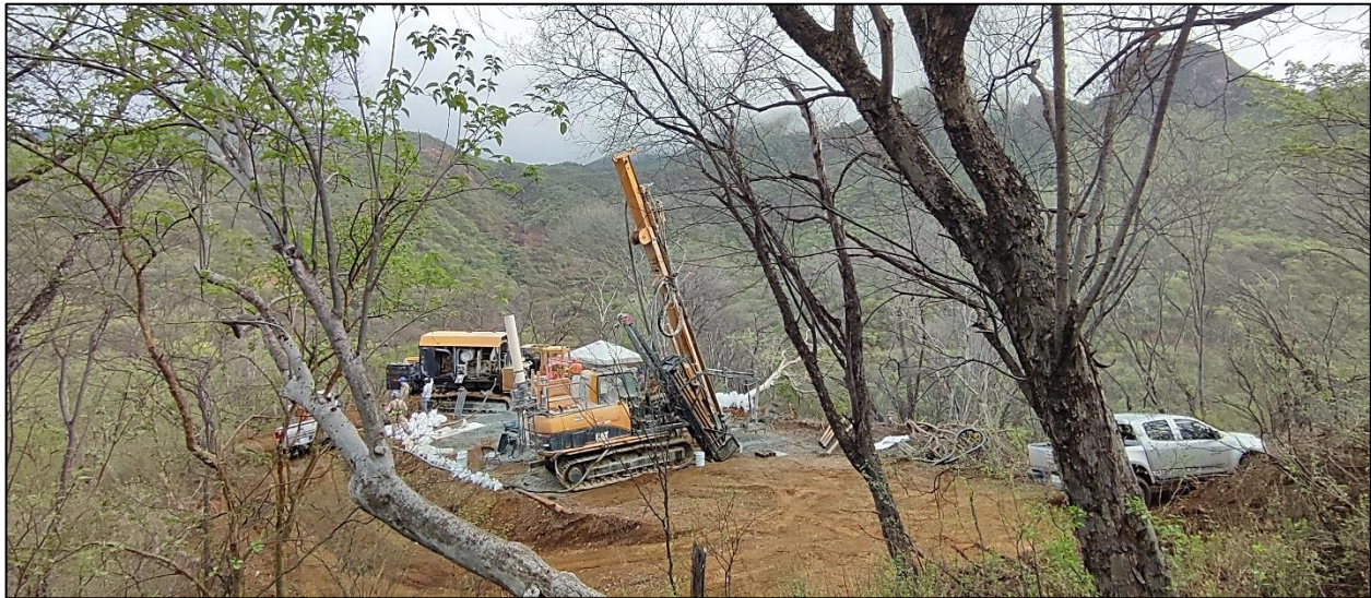
Figure 2. Minera Drilling on DIA22-09 at PAD #46 above and southwest of the historical mine workings at El Pillado target.
